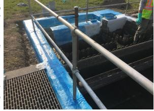
the crew applied a thin coat of Mainstay DS-5 100% Solids Epoxy Coating. The fiberglass reinforcement was then installed using fiberglass mat and cloth laid onto the wet epoxy and saturated with Madewell 1312E Epoxy Saturant. The material was left to cure overnight.
